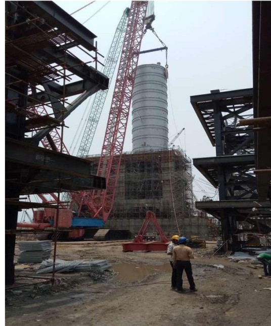
Assembly, Erection and installation of Heater Unit, Panipat, Haryana
