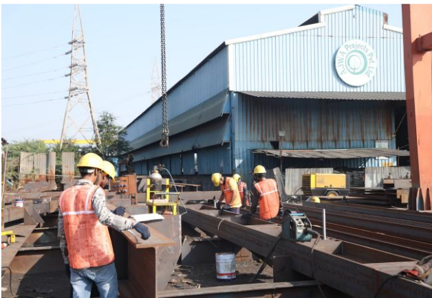
Welding and Grinding Area
