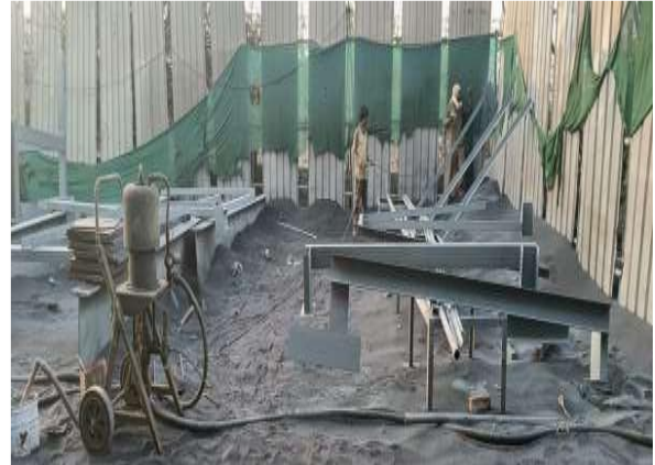
Blasting & Priming Area
