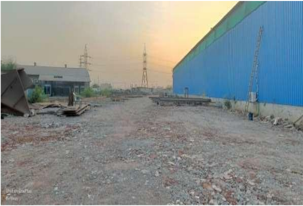
Open Fabrication Yard
