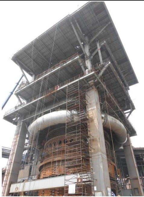
Erection of Blast furnaces at Dolvi, Maharashtra
