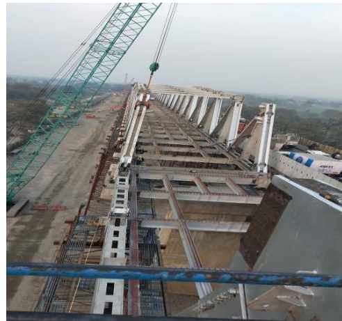
Assembly of pre-fabricated structure, Jammu and Kashmir
