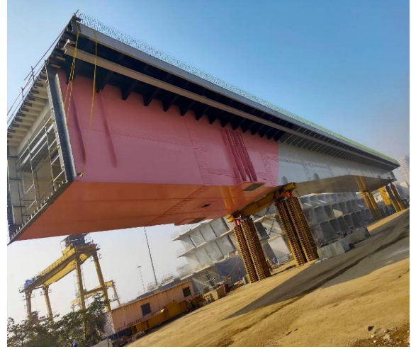
Steel Deck for bridge, at Sewri, Maharashtra
