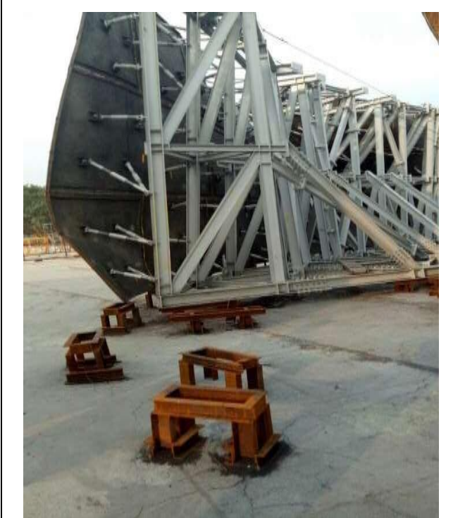
Steel Fabrication and Erection work at Kevadia, Gujarat
