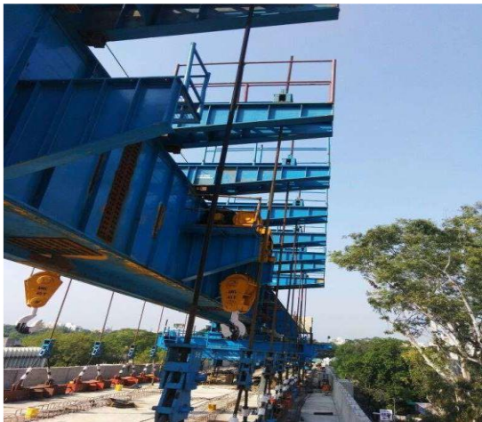
Launching of Precast module for Metro Project, at Nagpur, Maharashtra
